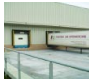
Loading Bay Equipment
